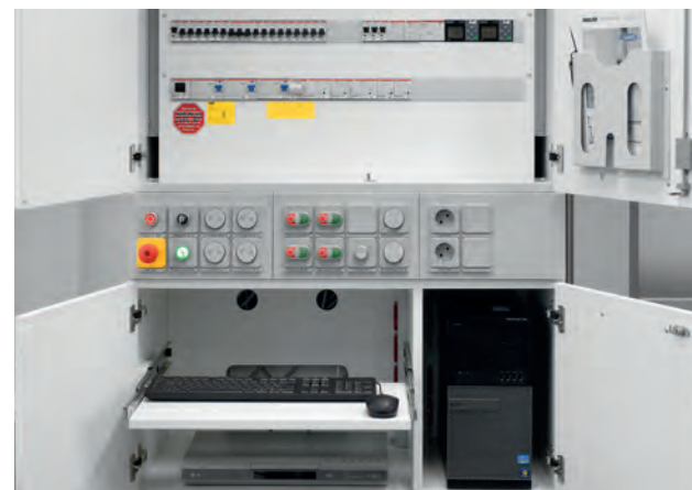
Top: electrical sub-distribution, Middle: integrated multimedia compartment
